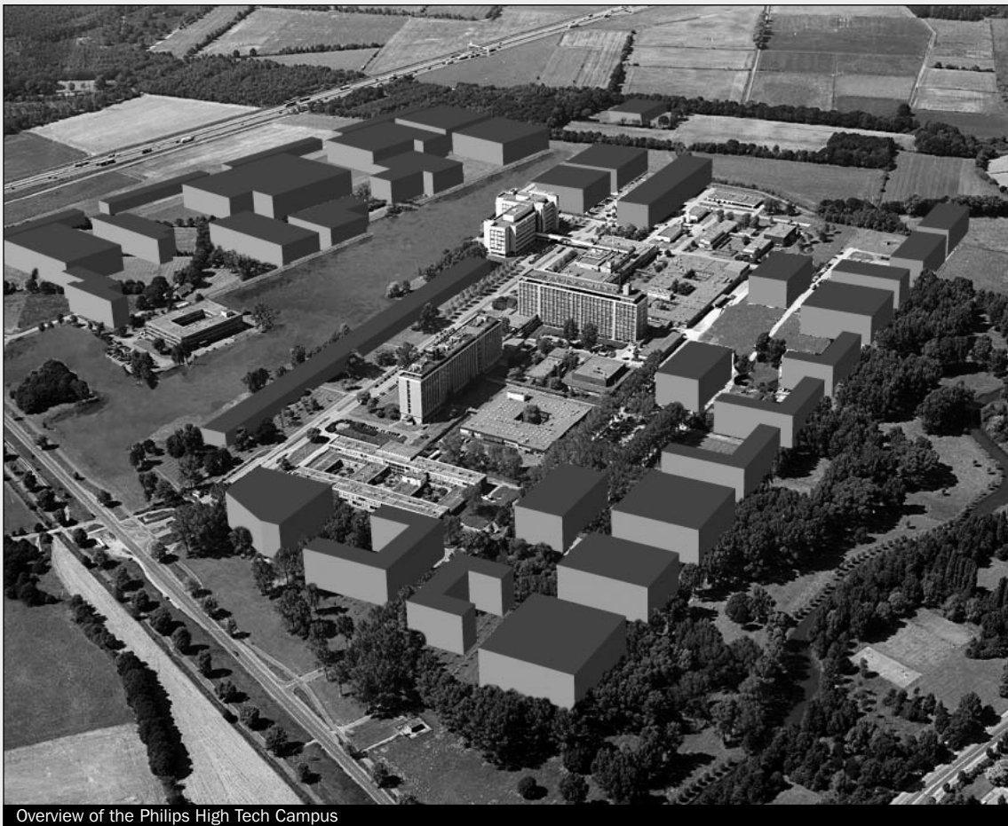
Overview of the Philips High Tech Campus
